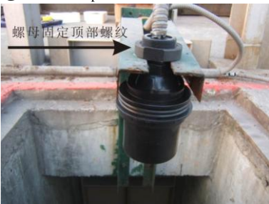
① fix the top thread with the nut
