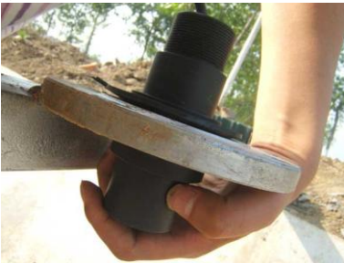
⑦ Screw the nut and fix the transducer
